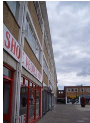
The Inland Revenue Building, Chequers Court – due for redevelopment
